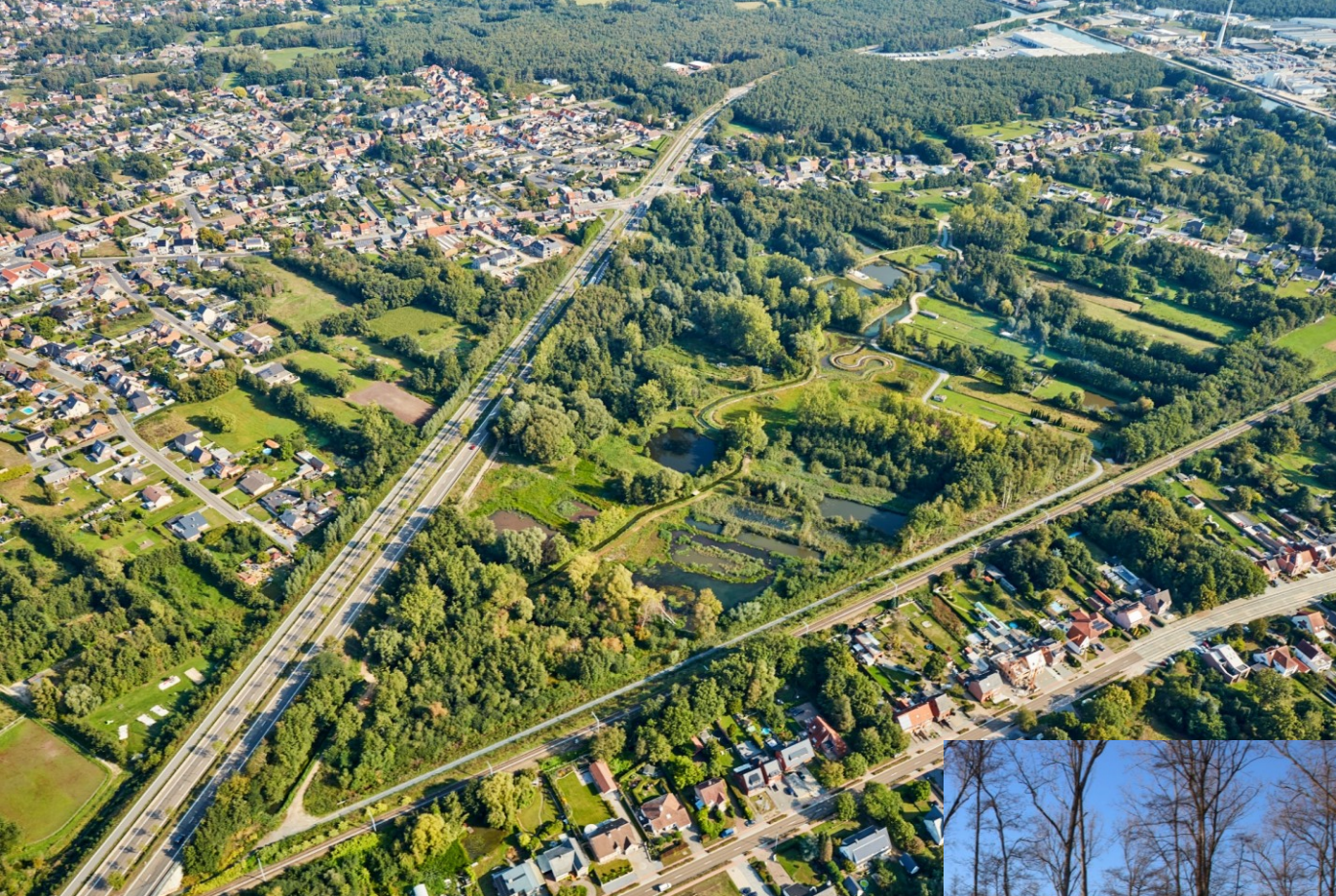
The floodplain upstream of Mol, after restoration works took place
